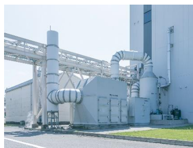
Deodorizing equipment (Itakura Facility)
